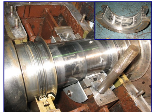
Identification of turbine front bearing failure on an 8 MW TG set at one of the sugar mill
